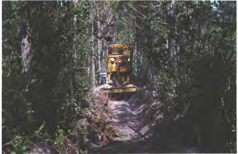
Establishing a control line in heavy rough
